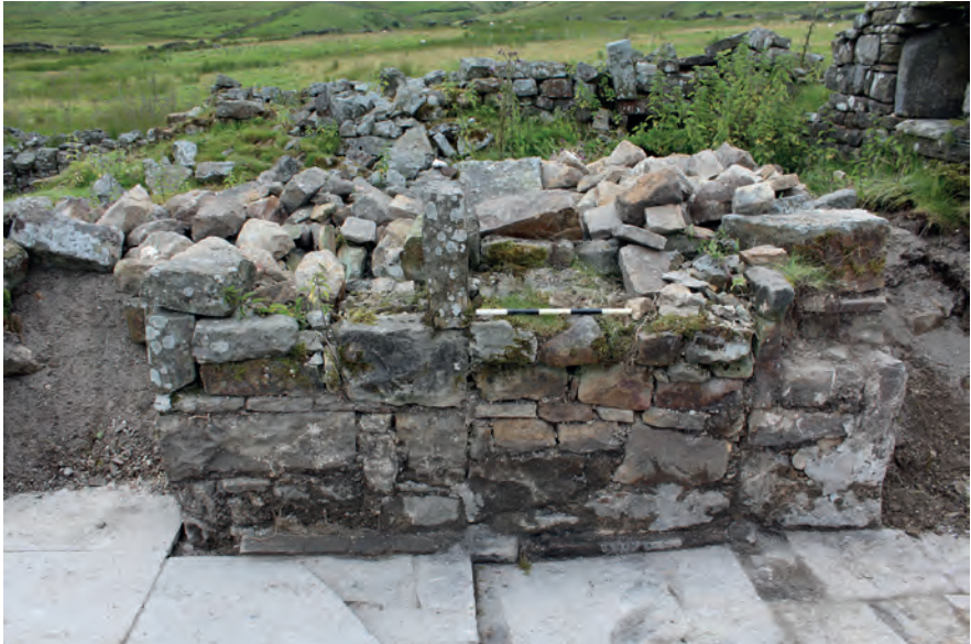
Figure 12 Central cross wall between Rooms B and C facing west. The openings to either end are visible, as is the blocked door positioned to the right of centre
