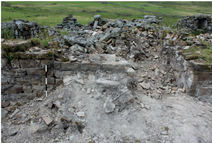
Figure 18 Partially cleared front (south) wall of Room A at the western end of the range. The width of the original cart entry can be seen in the straight join to the right of the scale bar
